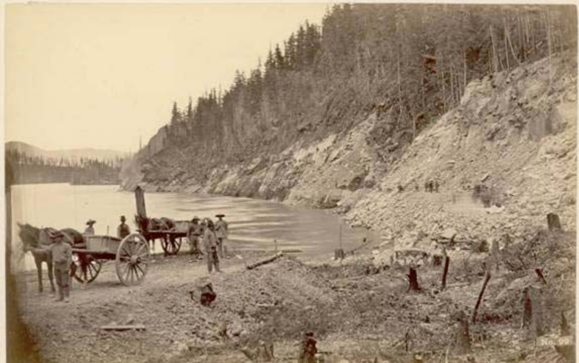
Figure 4.6: Chinese laborers grading near Heron, Montana, 1881. Courtesy of Denver Public Library.
